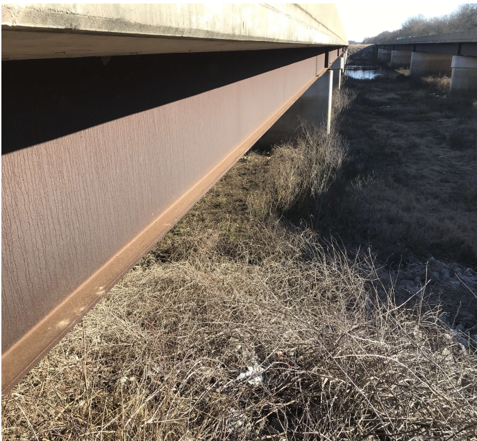
PHOTO 1 Description Small trees and vegetation are growing beside and under bridge.
